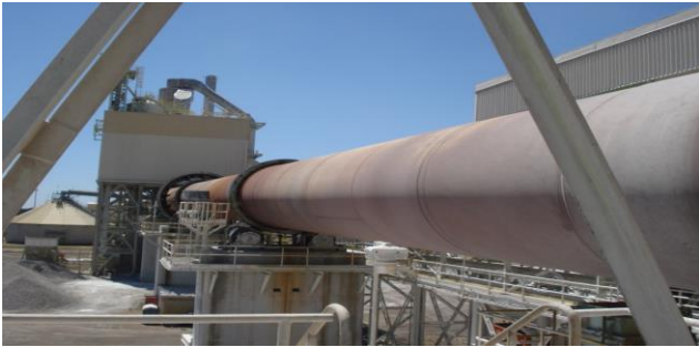
Rotary cement kiln looking towards the burning zone
